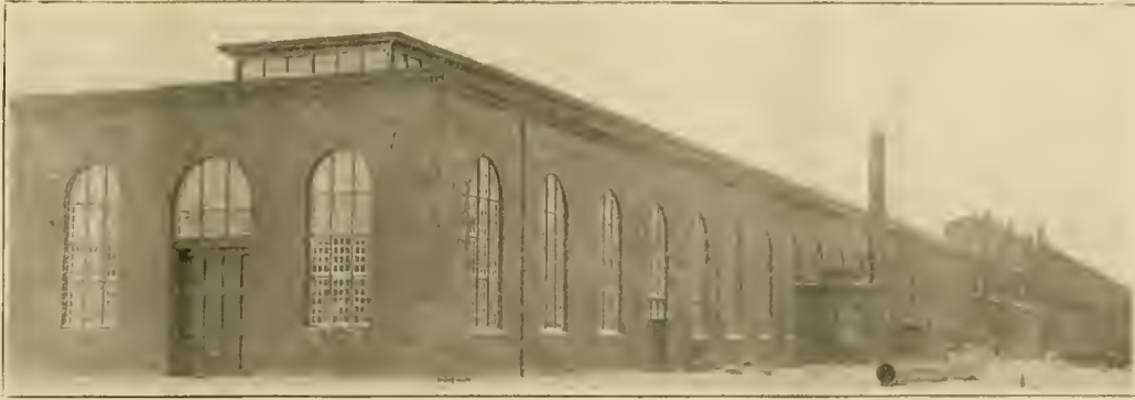
SMITH AND FORGE SHOP BUILDING, FROM SOUTHWEST CORNER, SHOWING FURNACE LEAN-TOS AND WASHROOMS AT RIGHT.
